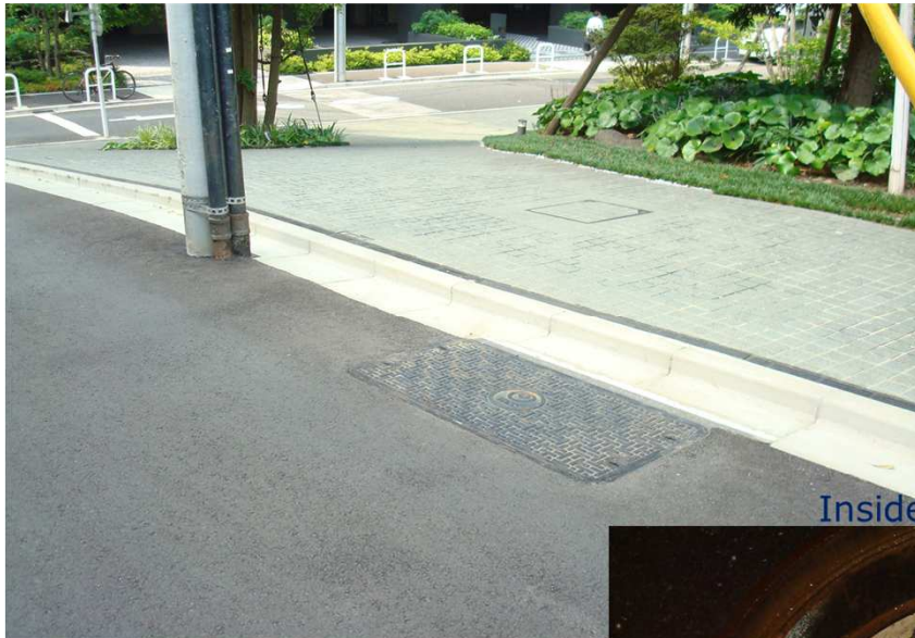
Handhole for Riser Point
